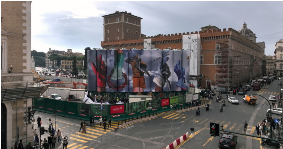
Photo Antonio Visceglia, Courtesy Webuild e Metro C.
